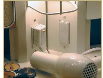
A rocker type light switch and 20 amp duplex outlet with built-in GFCI protection is mounted on the lower right side of the mirror frame.
